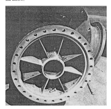
Vanes installed in submerged pump discharge line at Susquehanna station eliminated pump shaft vibration caused by flow turbulence.
